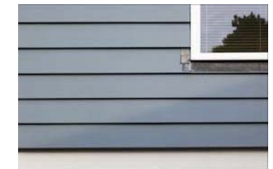
PROPOSED LAP SIDING: "EVENING BLUE" BY JAMES HARDIE, W/ WHITE FIBER CEMENT TRIM AT WINDOWS, TYP
