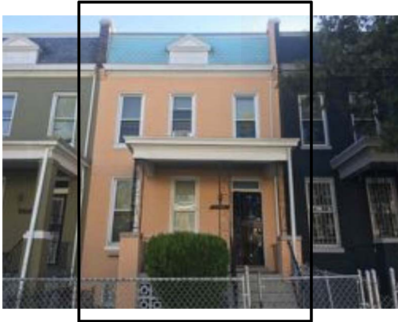
1135 MORSE ST. NE FRONT FACADE
