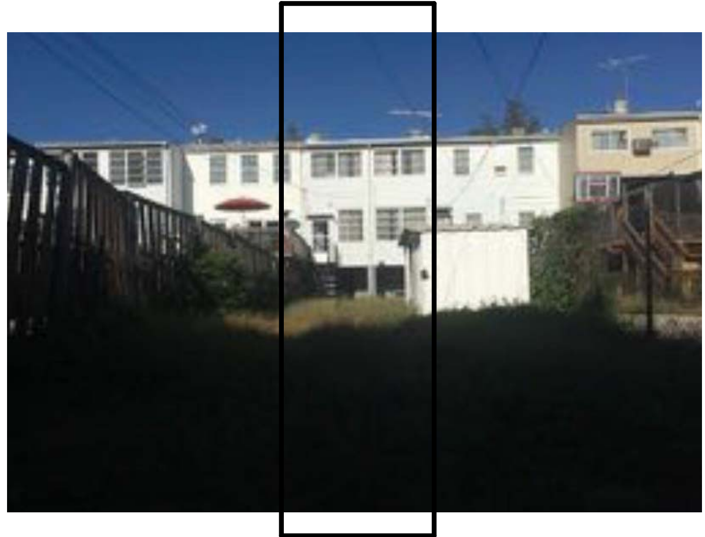
1135 MORSE ST. NE REAR FACADE
